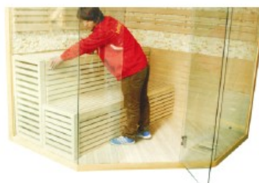
FIG-16 Assembling sitting board
