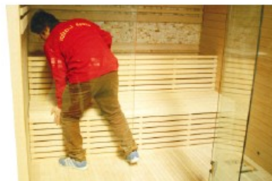
FIG-14 Assembling sitting board's support
