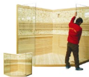
FIG-6 Assembling the glass window(Right)
