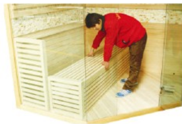
FIG-14 Assembling sitting board
