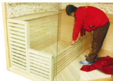
FIG-13 Assembling sitting board's support
