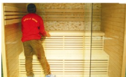
FIG-15 Assembling sitting board
