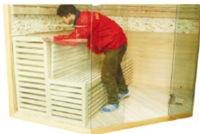
FIG-15 Assembling sitting board's support
