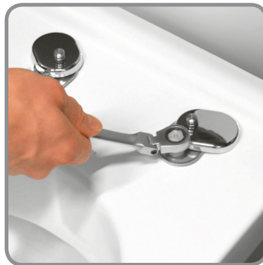
Tighten with Spanner
