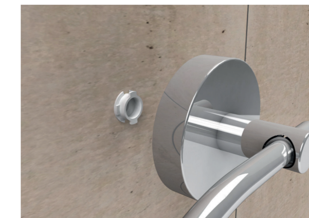
Positioned the alignment guide in desired location.
