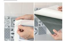
Peel away white backing paper (leaving the clear membrane in situ).
